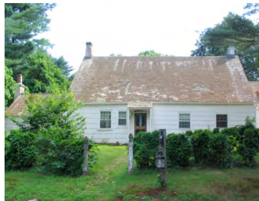
Figure 13. View of Barnswallow original house east façade showing fresh paint, new gutters, and wood shingle roof, 2005.
