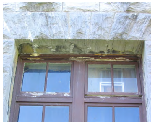
Figure 22. Detail of stable building window showing efflorescence and gypsum crust at lintel, 2005.
