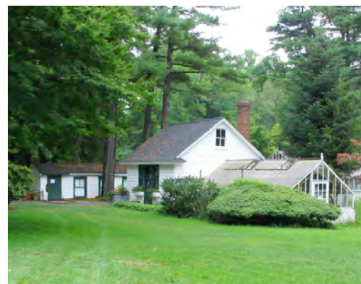
Figure 47. View of Bailey estate greenhouse looking north east, 2005.
