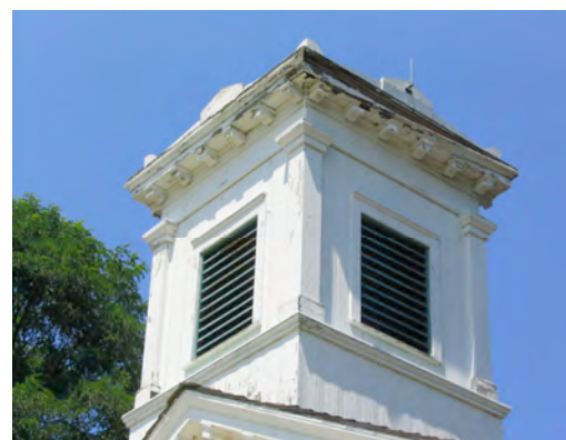
Figure 54. detail view of the Manetto Hill Church bell tower showing collapsing soffit and eave at north east corner, 2005.
