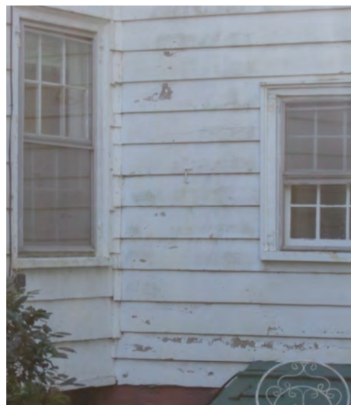
Figure 15. detail of the Malcolm House rear (east) façade showing peeling paint and mildew, 2005.
