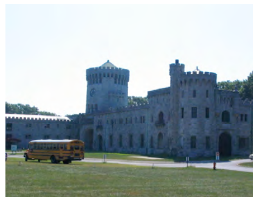
Figure 21. View of Castlegould showing the north and west facades, 2005.
