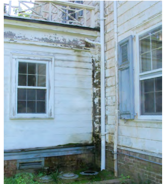
Figure 10. Detail of the east façade juncture between the main house and flat roof addition showing mold and algae growth due to a failed gutter system, 2005.
