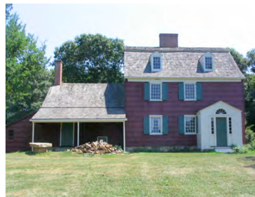
Figure 53. View of Hewlett House showing freshly painted west façade, 2005.
