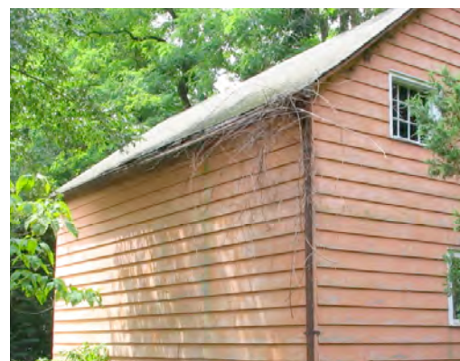
Figure 41. View of Elderfields barn east façade showing detached gutter and damaged fascia, 2005.
