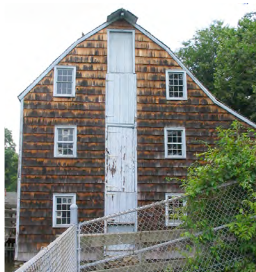
Figure 56. View of Saddle Rock Grist Mill west façade showing paint deterioration and damaged window glass, 2005.
