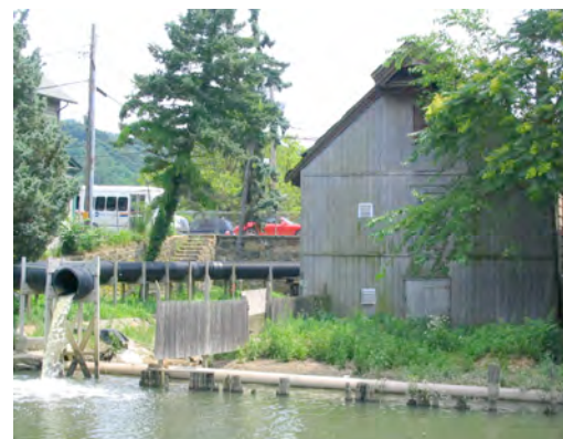
Figure 57. View of Roslyn Grist Mill north façade showing interim water diversion system, 2005.
