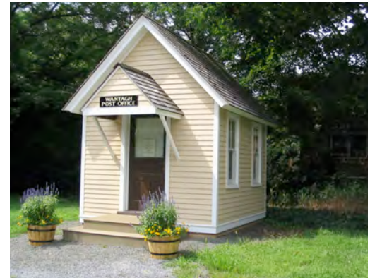
Figure 60. View of Train Museum Post Office south east corner showing completed restoration, 2005.
