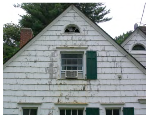
Figure 46. View of Bailey estate stables east façade showing deteriorated paint and damaged trim, 2005.
