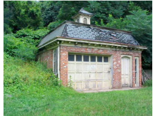
Figure 50. View of Cedarmere garage south façade showing overall advanced deterioration, 2005.
