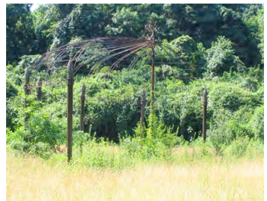
Figure 7. View of the west side Chelsea game court showing rusting gazebo and overgrown plant material, 2005.
