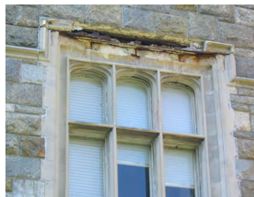
Figure 23. View of typical hempstead House window showing deteriorated lintel masonry and exposed, rusting support member, 2005.
