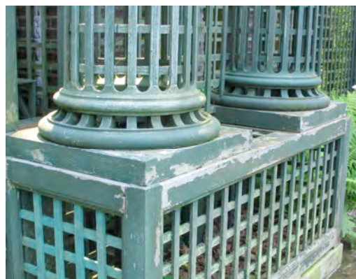
Figure 34. Detail view of Clayton estate trellis showing paint loss, 2005.
