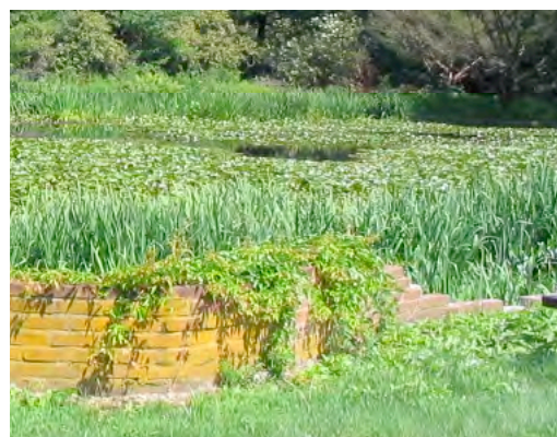
Figure 4. View of the Chelsea lotus pond and serpentine wall showing damaged masonry at the right, 2005
