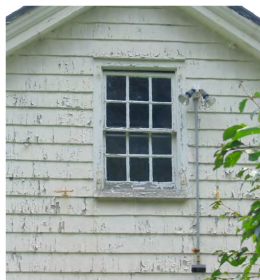
Figure 39. Detail view of Elderfields west façade showing paint failure, 2005.
