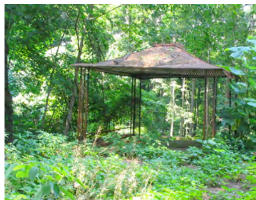
Figure 36. View of the Dewy House iron gazebo looking north showing severe rust and general deterioration, 2005.
