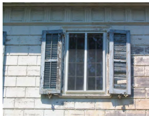
Figure 9. Detail of Nassau Hall west façade showing bear wood and damaged shutters, 2005.
