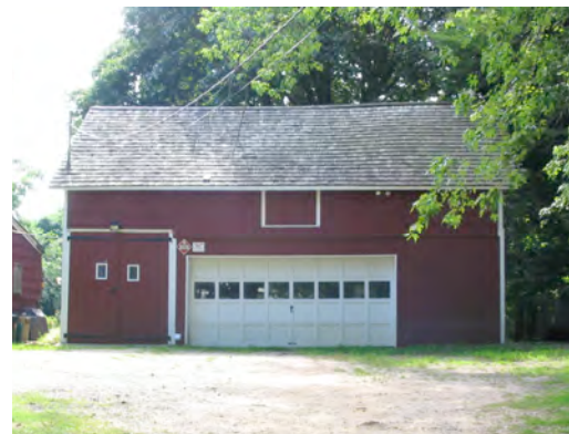
Figure 17. View of the Malcolm carriage house showing new paint, good roof, and dry foundation, 2005.
