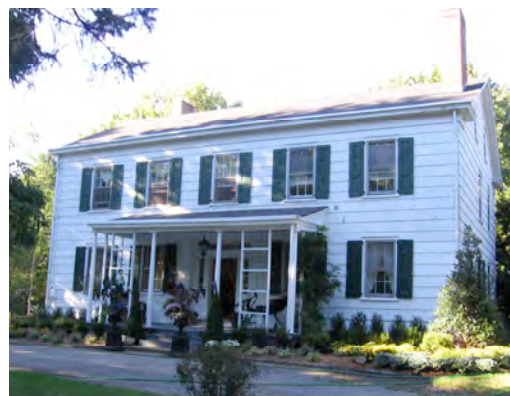
Figure 14. View of the Malcolm House south façade, 2005.
