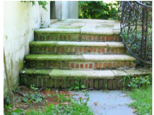
Figure 5. Detail of Chelsea north façade west wing staircase showing continued drainage issues and algae growth, 2005
