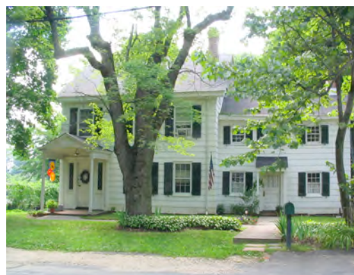
Figure 20. View of the Coles House east façade, 2005.
