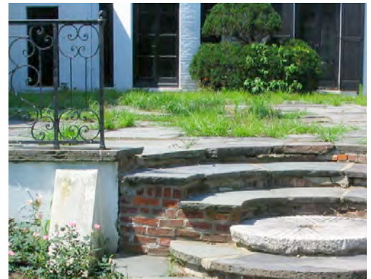
Figure 6. View of garden façade paving showing loose mortar and masonry as well as volunteer grass at the patio, 2005
