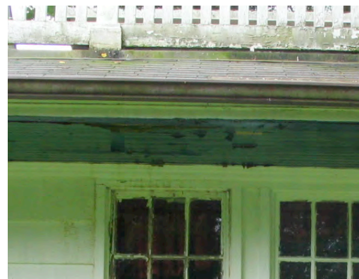
Figure 45. Detail view of Bailey main house north façade overhanging roof showing water damage at soffit and window, 2005.
