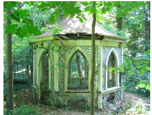
Figure 11. View of the Nassau Hall gazebo before Eagle Scout repair showing damaged lattice and corroded metal roof, 2005.
