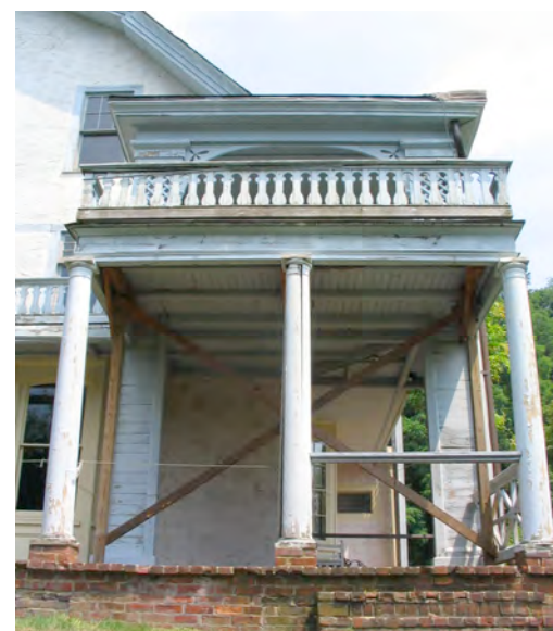
Figure 49. View of Cedarmere west façade showing stabilized porch, 2005.
