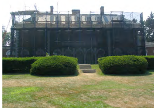
Figure 33. View of Clayton east façade showing scaffolding set for exterior repairs, 2005.
