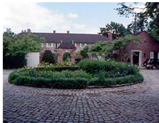
Figure 26. View of Mille Fleurs west façade, 2001.
