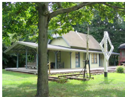
Figure 58. General view of the Wantagh Train Museum looking south west, 2005.
