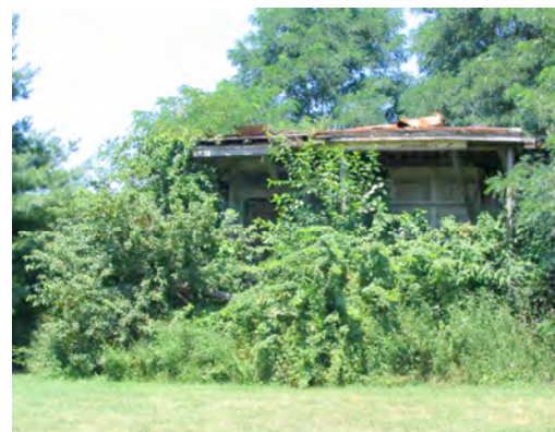
Figure 55. View of non-restored structure located west of the Manetto Hill Church, 2005.
