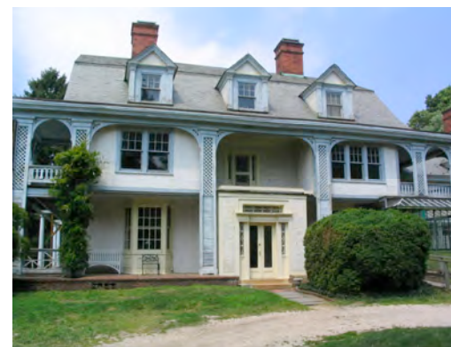
Figure 48. View of Cedarmere south (main) façade, 2005.
