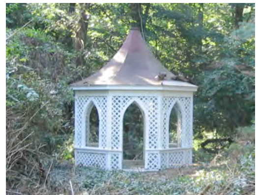
Figure 12. View of Nassau Hall gazebo after Eagle Scout repair showing new lattice, fresh paint, and metal roof awaiting restoration.
