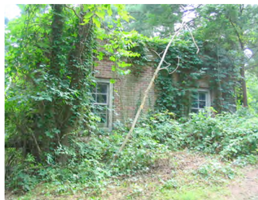
Figure 30. View of typical Welwyn out building showing excessive overgrowth and subsequent deterioration, 2005.
