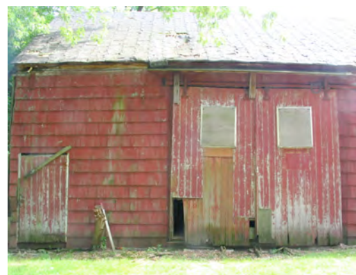
Figure 16. View of the Malcolm barn north façade showing a state of overall deterioration, 2005.
