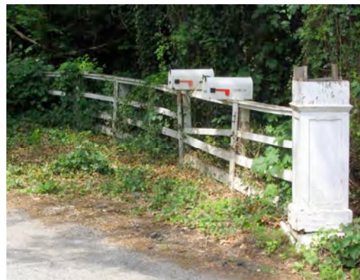
Figure 43. View of Elderfields main entrance gate post showing lost urn finial, 2005.
