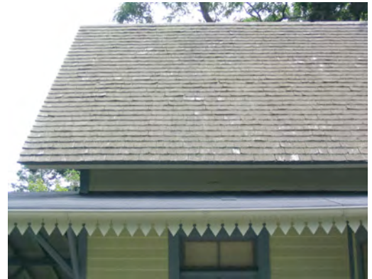
Figure 59. Detail View of Train Museum north façade showing new gutters and flat asphalt roof, as well as wood shingle sloped roof, 2005.
