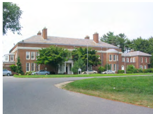
Figure 27. View of Welwyn main house, south façade, 2005.
