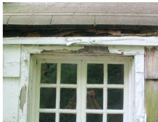
Figure 38. detail view of Elderfields south façade single story bump out showing significant damage at eave and window sill, 2005.
