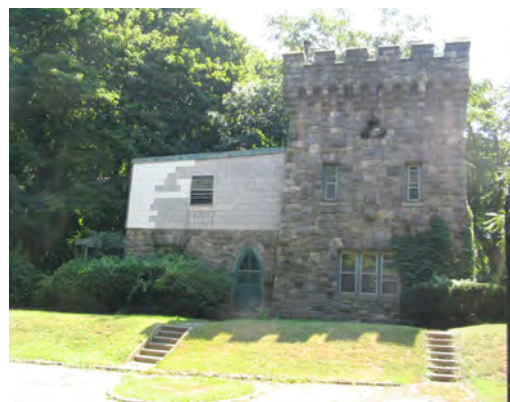
Figure 25. View of the main gate house north façade showing inappropriate second floor addition, 2005.
