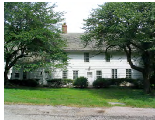
Figure 37. View of Elderfields south (front) façade, 2005.
