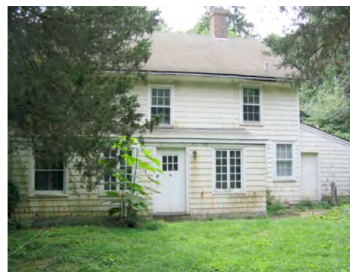
Figure 40. View of Elderfields north façade, west side showing algae growth at lower level and damaged gutter above, 2005.
