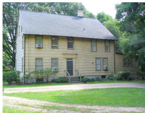
Figure 18. View of the Elias Hicks House front (north) façade showing an aged roof, 2005.
