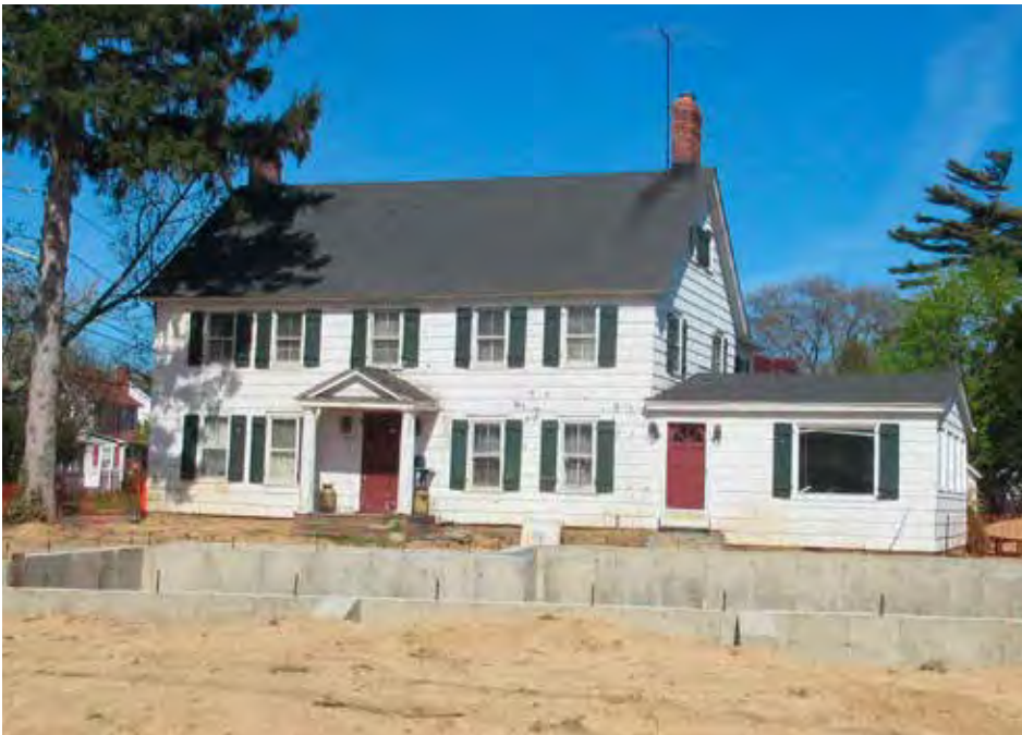
New lots were redeveloped adjacent to the Smith House, pictured above in 2016. (Courtesy of the Home In Babylon blog)
