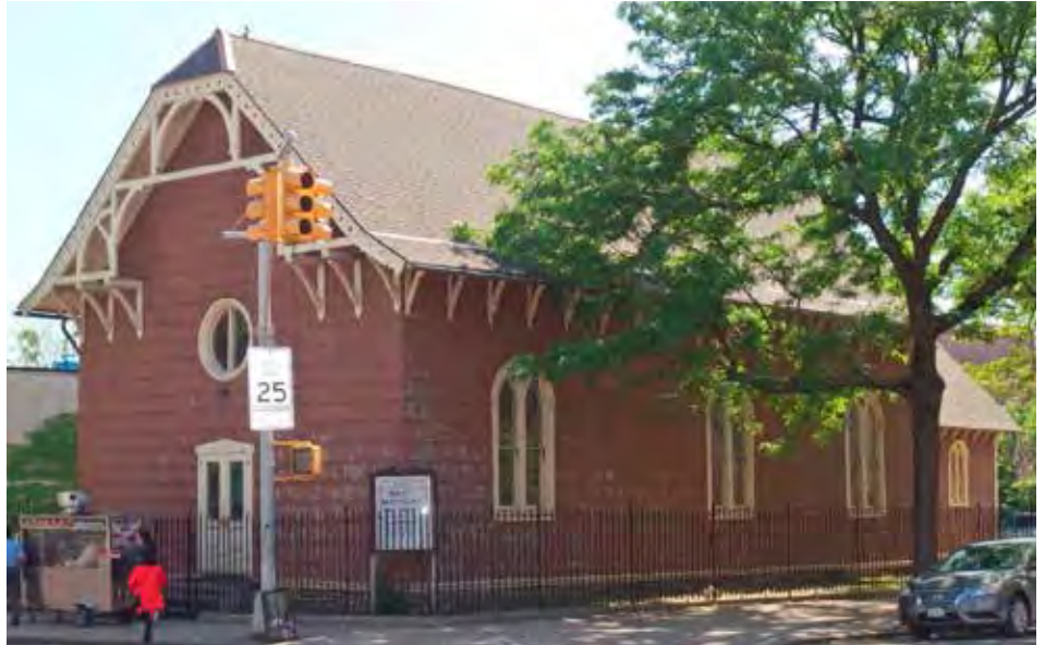
Old Saint James Episcopal Church, 2017. Today’s exterior of Old Saint James Church is the result of a major remodeling in 1883. The Gothic Revival and Stick style features were most likely added at the same time. These included the truss-like trim below the clipped gable ends, overhanging eaves with brackets, the round window, and drip molding. (Courtesy of Marianne Hurley)
