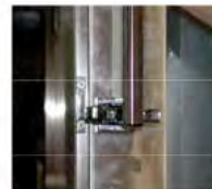
Door Latch Too Low
