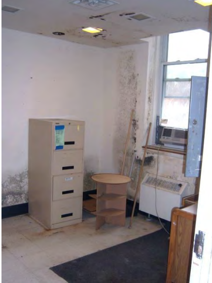
Existing water and mold found on second floor at areas of roof leaks. UPDATE: The existing owner reports that this area has continued to leak, but some furniture and soft goods have been removed.
