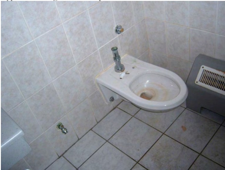
Typical damage from vandalism, removed plumbing fixtures and accessories. In many areas exposed pipes have been removed on the second floor.
