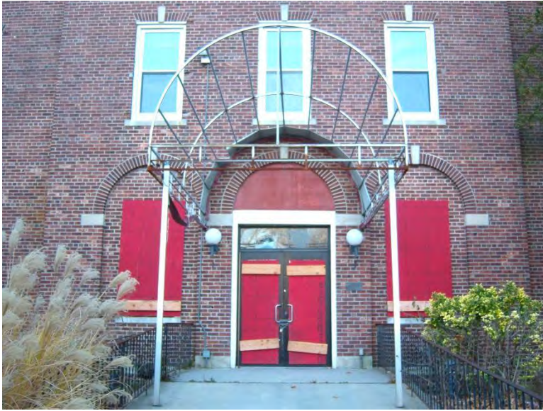
Existing main entrance
