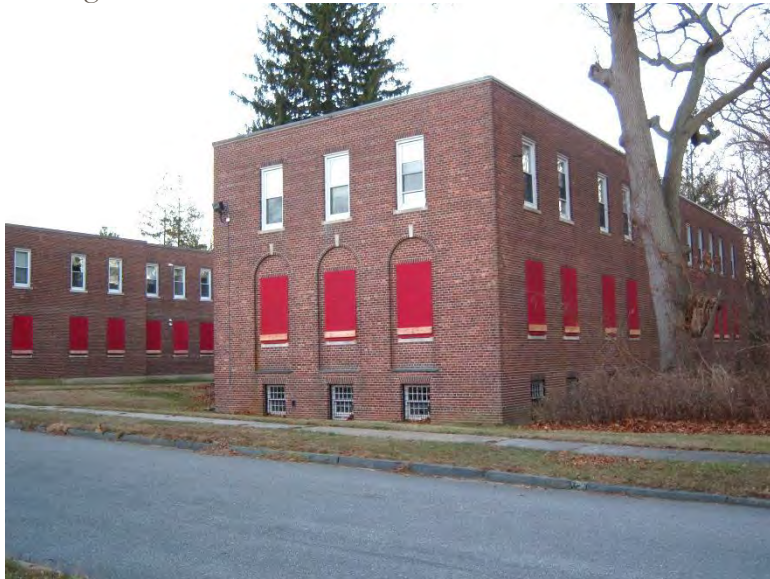
Existing site landscape and large trees
