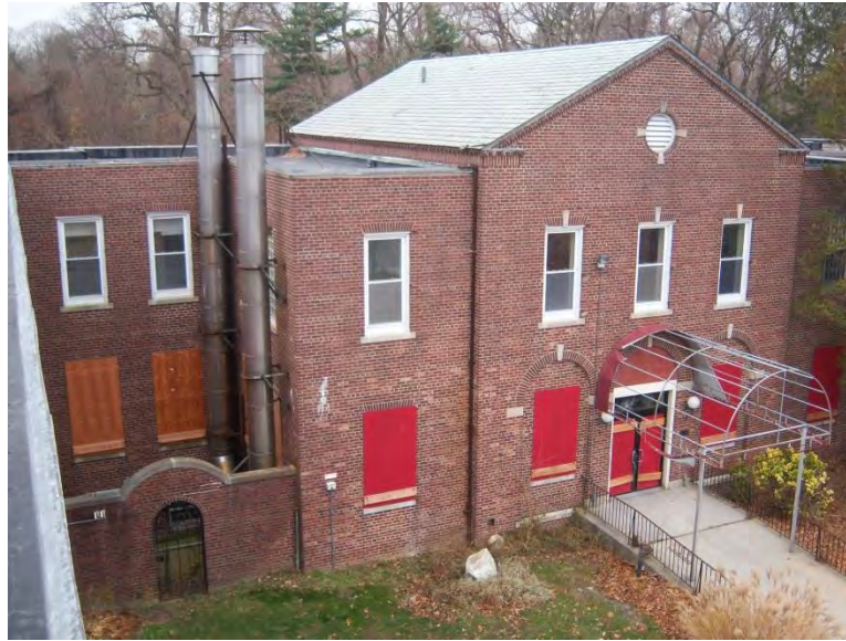
Existing building 1 canopy
