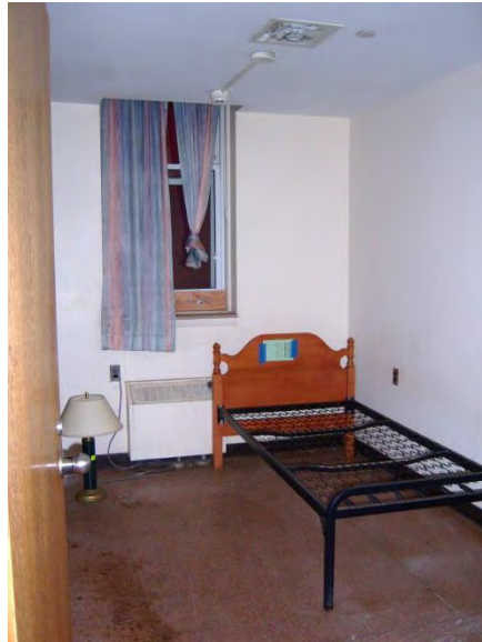
Existing room with terrazzo flooring
