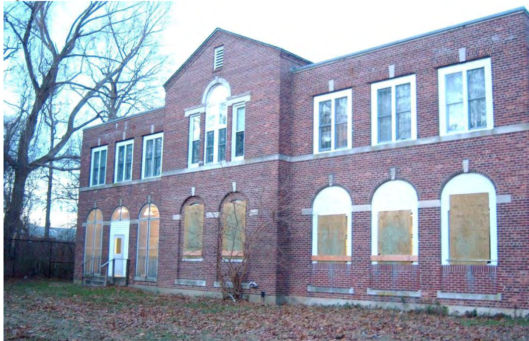
Rear of Building 1 showing wood/steel handrails
