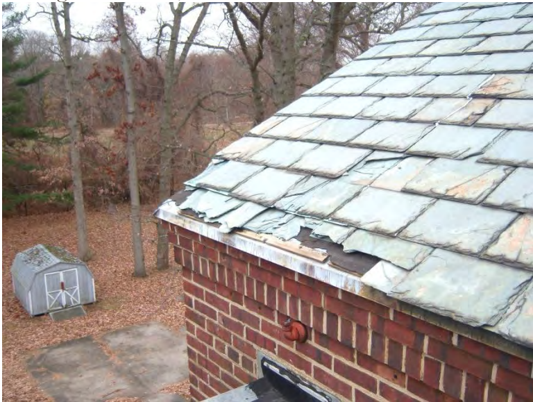
Existing slate roof damage
