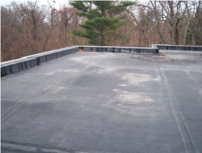
Existing EPDM roof, note the multiple insulation failures
