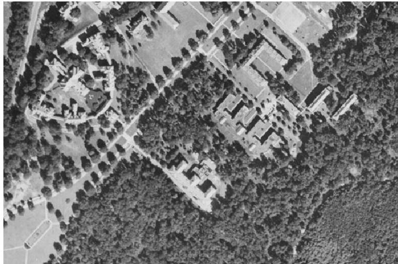
Kings Park PC Circa 1952 with Building 1 in the Center and Building 2 (bottom demolished)
