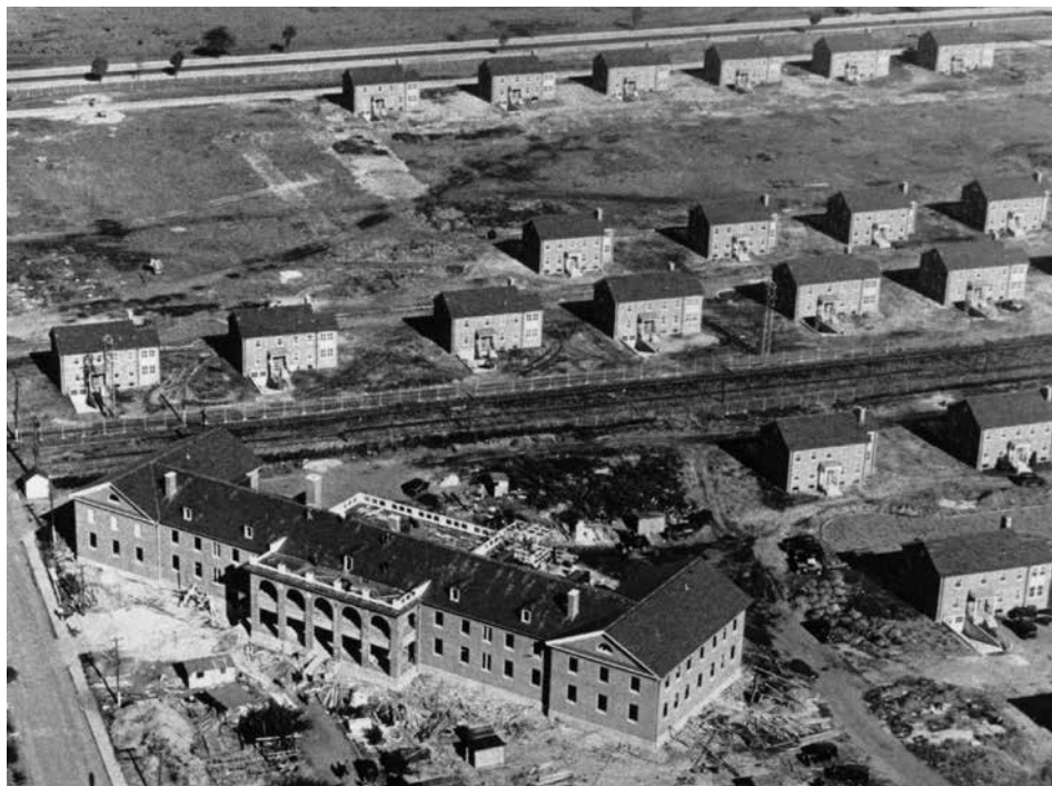
Mitchel Field, October 31, 1932 (Courtesy of the Cradle of Aviation Museum). Aerial view of the Bachelor Officers Quarters and surrounding area under construction.
