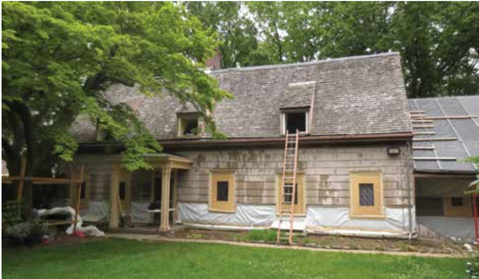
Bowne House under construction, 2014 (Photo courtesy of Jan Hird Pokorny Associates).
