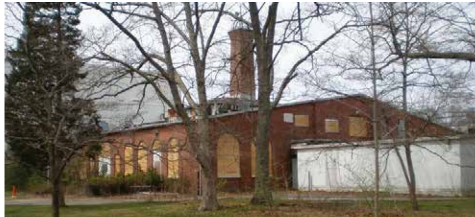
Volunteers have been working to clean up the site since the Science Center purchased the property in 2012.
