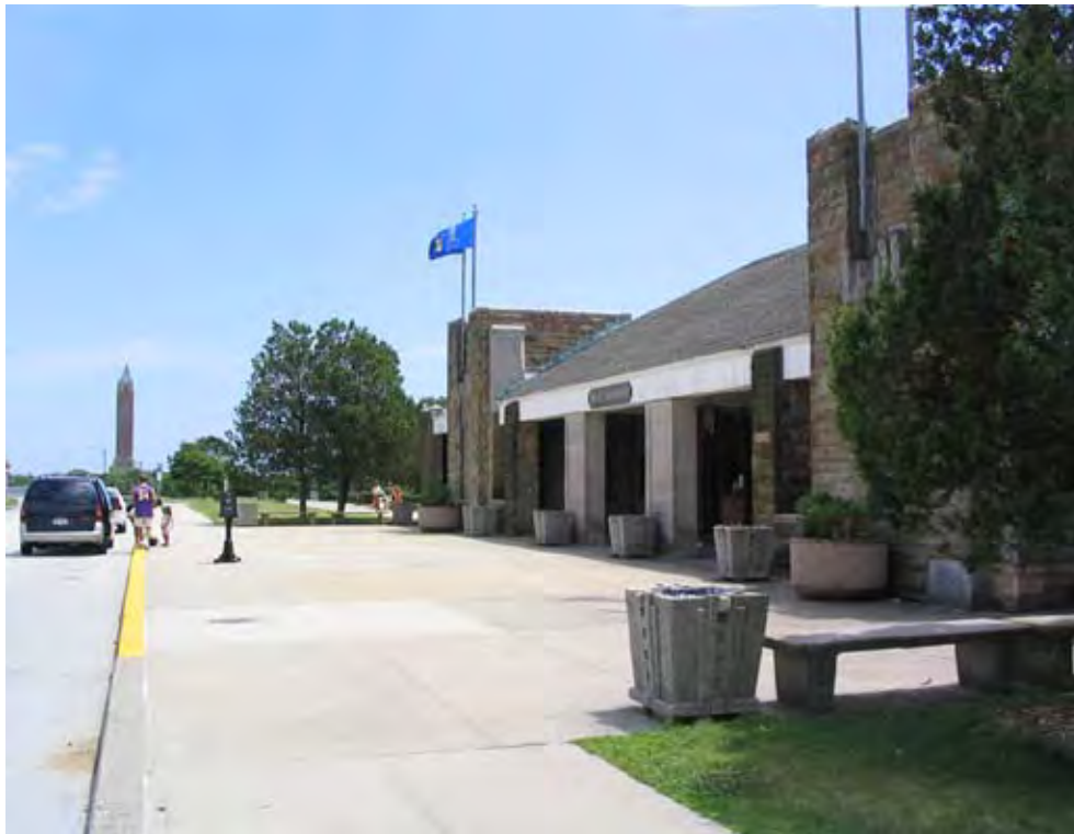
Figure 42: West Bathhouse north facade showing removed landscaping, altered cornice, and original Art Deco planters used for garbage, 2004.
