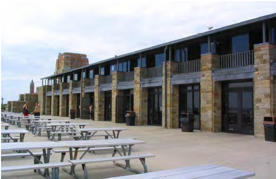
Figure 32: East Bathhouse south facade showing replacement materials, 2004. What was once a simple yet charming building is made dreary by the cold utilitarian quality of the new materials. Artistically carved wooden posts, balustrade, and doorways are replaced by flat, lifeless aluminum components, and corrugated fiberglass replaces the colorful canvas awning. Even the aluminum picnic benches seem mean compared to the inviting cluster of round tables, chairs, and canvas umbrellas.
