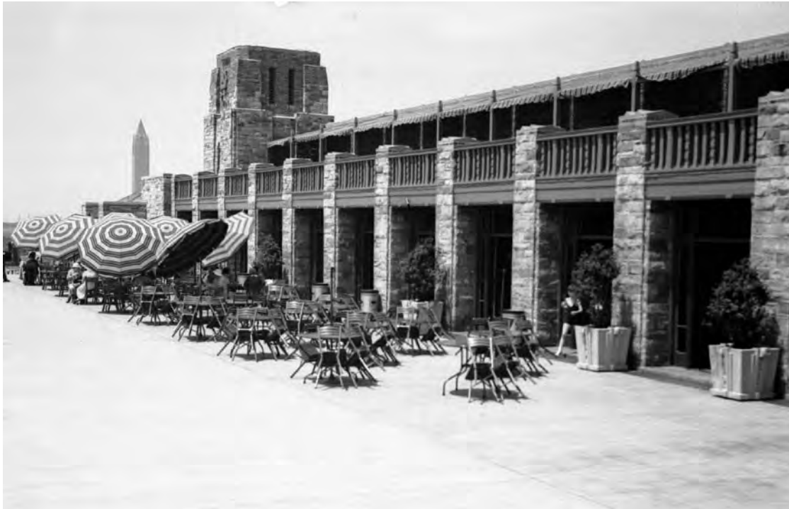
Figure 31: East Bathhouse south facade showing original observation deck with wooden posts and balustrade, canvas awning, and patio planters, 1935. ( New York State Office of Parks, Recreation, and Historic Preservation, Long Island Region )
