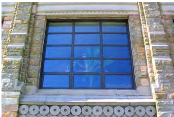
Figure 6: Replacement second floor West Bathhouse metal window, 2004. The new aluminum frames are flat, have no construction details, and do not adequately address the character of the originals.
