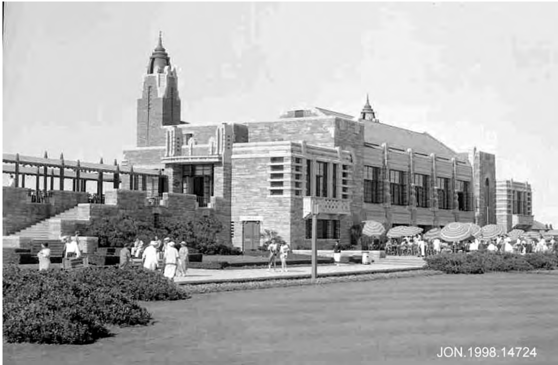
Figure 44: West Bathhouse south facade showing original landscape, towers, cast-stone trim, and canvas awnings over second level walkways (center left), 1931. ( New York State Office of Parks, Recreation, and Historic Preservation, Long Island Region )
