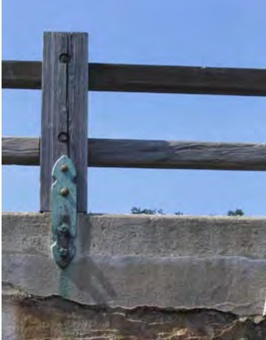
Figure 24: Original hardware remaining at Ocean Parkway underpass, 2004. (Note deteriorated concrete.)
