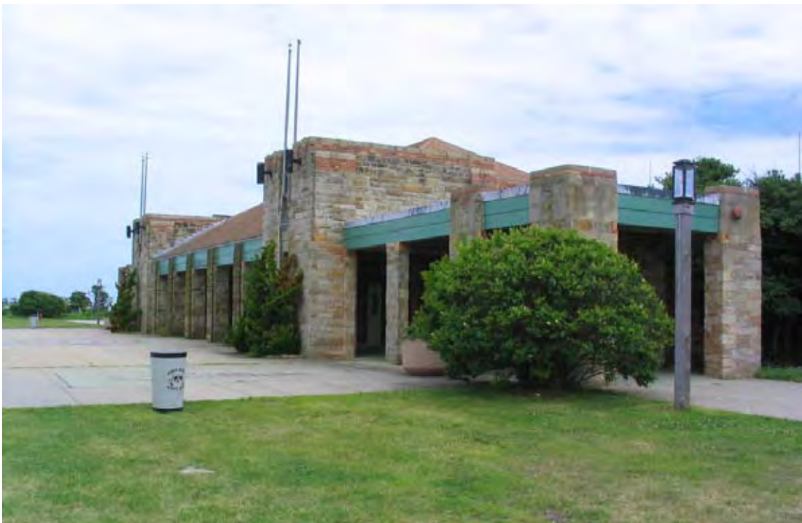
Figure 28: East Bathhouse north facade showing removed rooftop lights and brackets, and reduced landscape, 2004.
