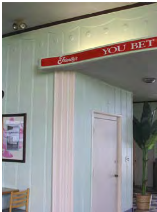
Figure 56: West Bathhouse former Marine Dining Room looking south, 2004. The original wall details have been replaced by vertical wood paneling, the entryway columns have been removed, and a drop ceiling reduces the interior space. In addition, a partition wall divides the former dining area in two.
