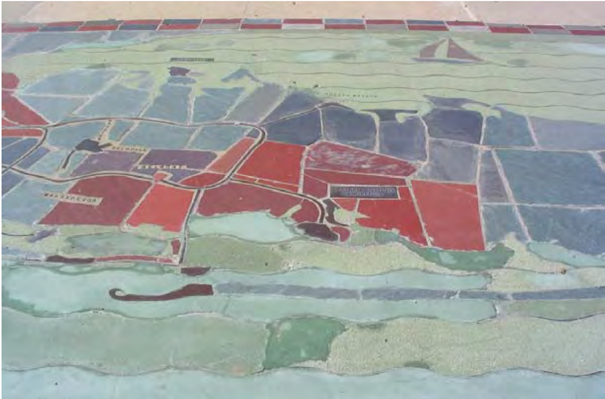
Figure 37: Detail of mosaic map of Long Island at north side of Central Mall showing poorly matched concrete repair, 2004.
