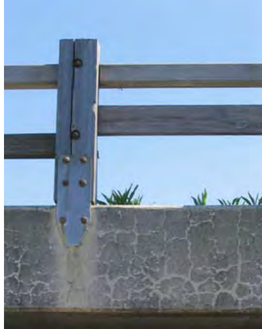
Figure 25: Replacement hardware at Ocean Parkway underpass, 2004. (Note misaligned cross members.)
