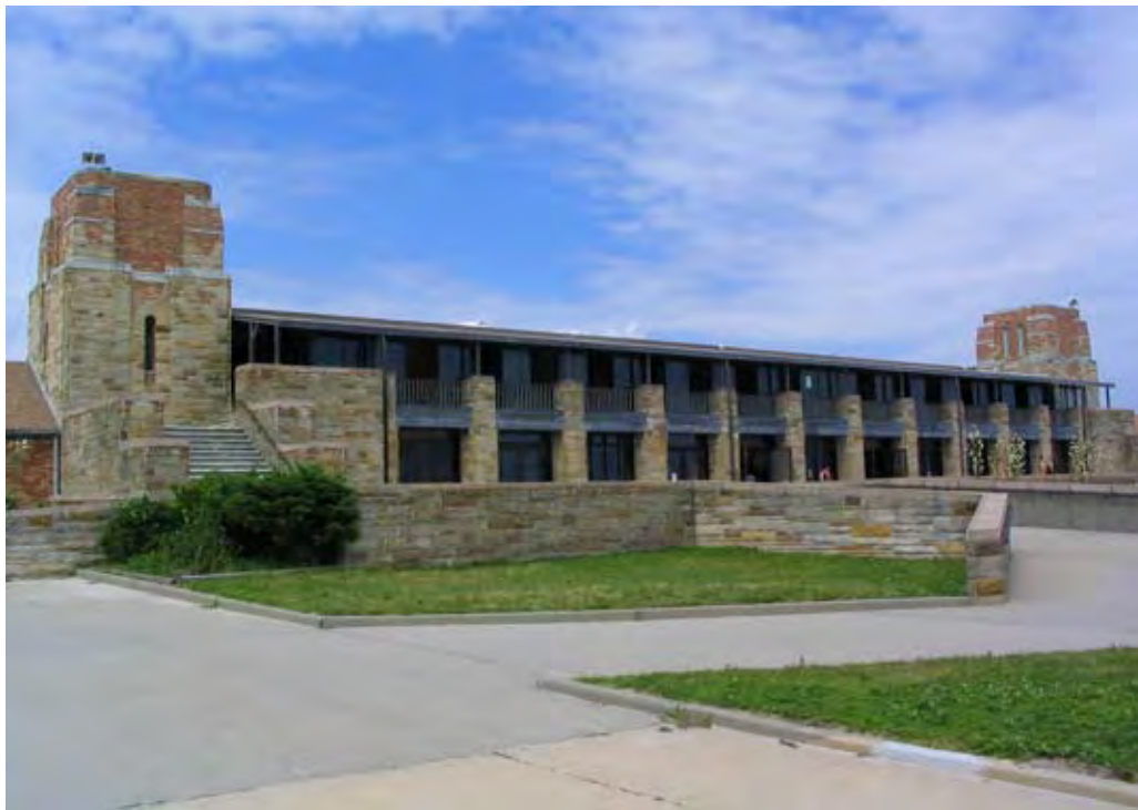
Figure 30: East Bathhouse south facade showing a building devoid of its original embellishments, 2004. The landscape is reduced, the tower clocks are removed, replacement railings, doors, and awning are of cheaper materials, and handicap access ramp severs the patio retaining wall.
