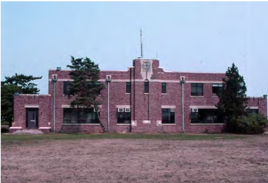
Figure 58: Police Headquarters south facade showing surviving decorative features and replacement windows, 2002. (Note: second floor replacement windows do not maintain the same unit ration as the originals: two units replace three in each fenestration.)
