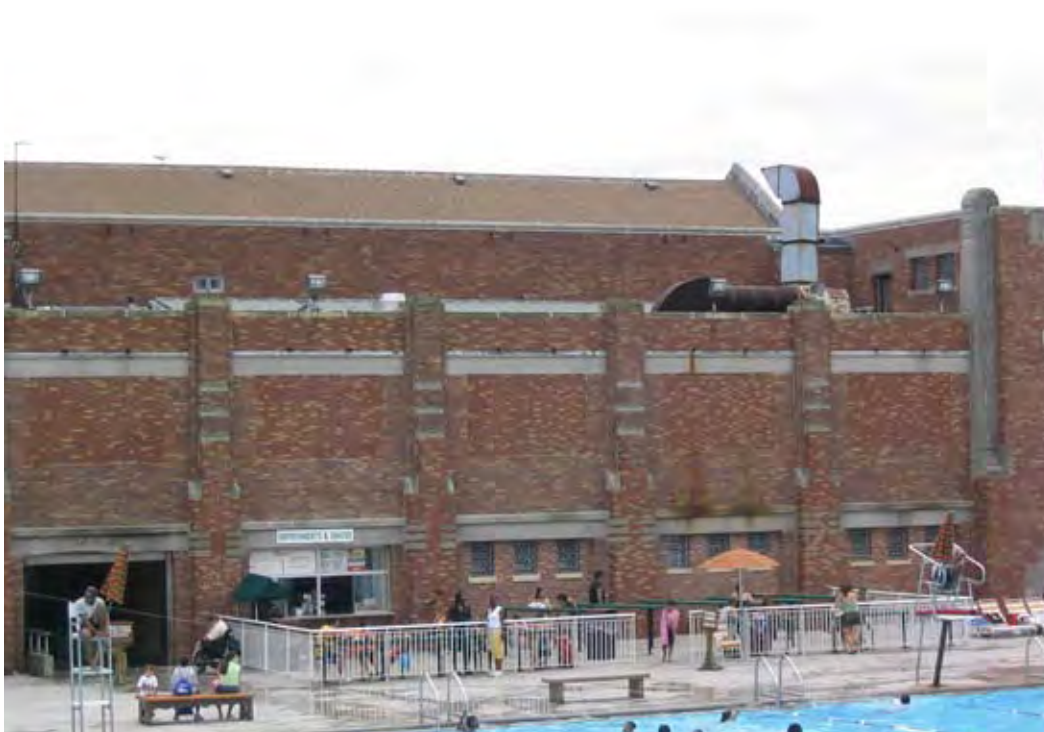
Figure 49: West Bathhouse pool area facing south showing filled windows, altered roof line, doorways and decorative grills, and removed cast-stone trim details, 2004.
