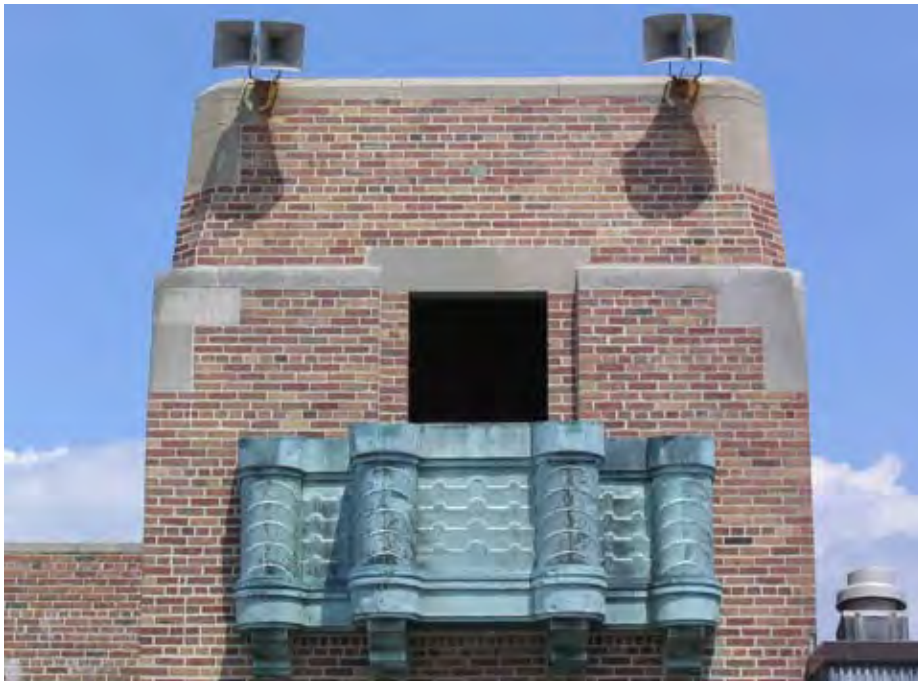
Figure 36: Central Mall Cafeteria south facade detail showing surviving original sculpted copper-clad balcony, 2004.
