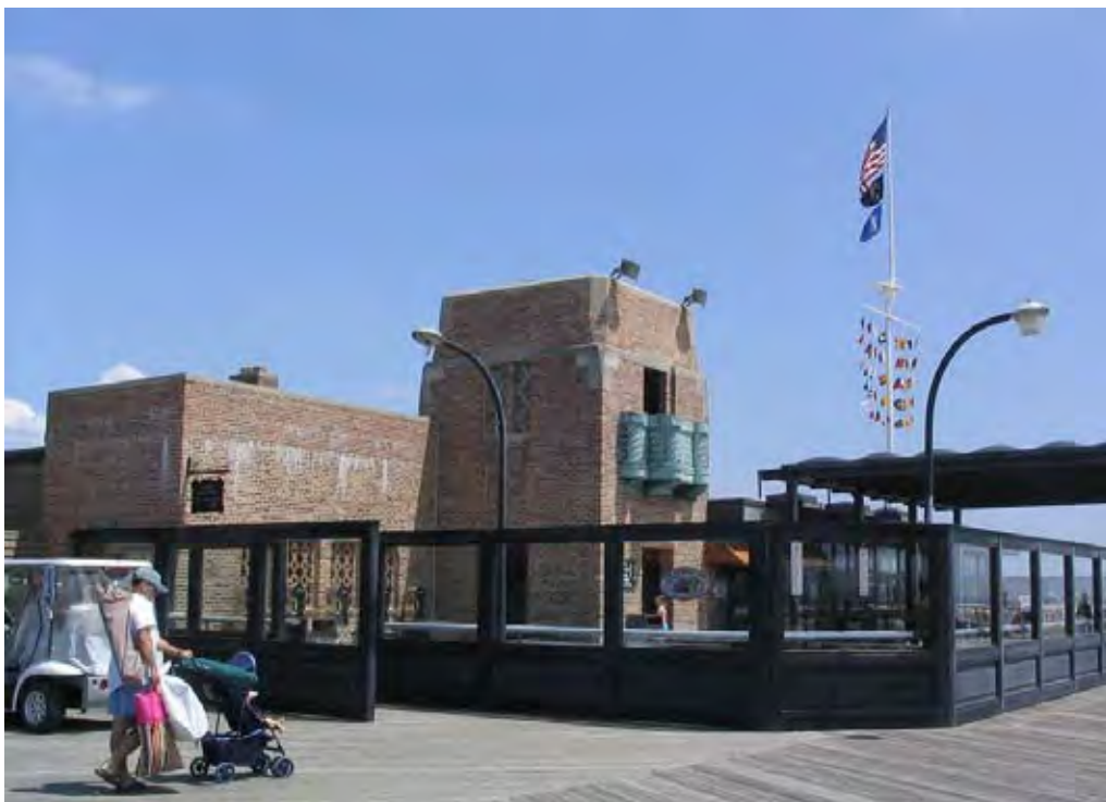
Figure 43: Central Mall Cafeteria south facade showing windscreen addition and removed stairway and observation deck, 2004.
