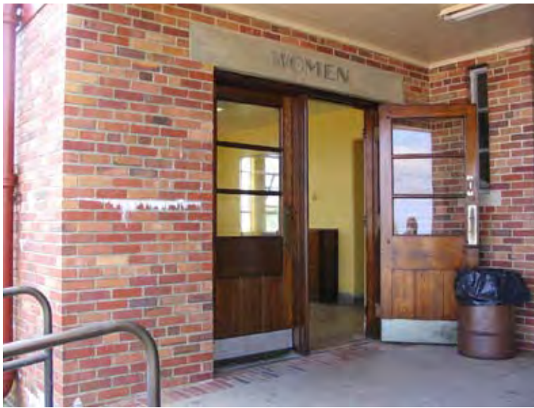
Figure 63: Zach's Bay comfort station showing original signage, wooden doors, and deteriorating mortar joints, 2004.
