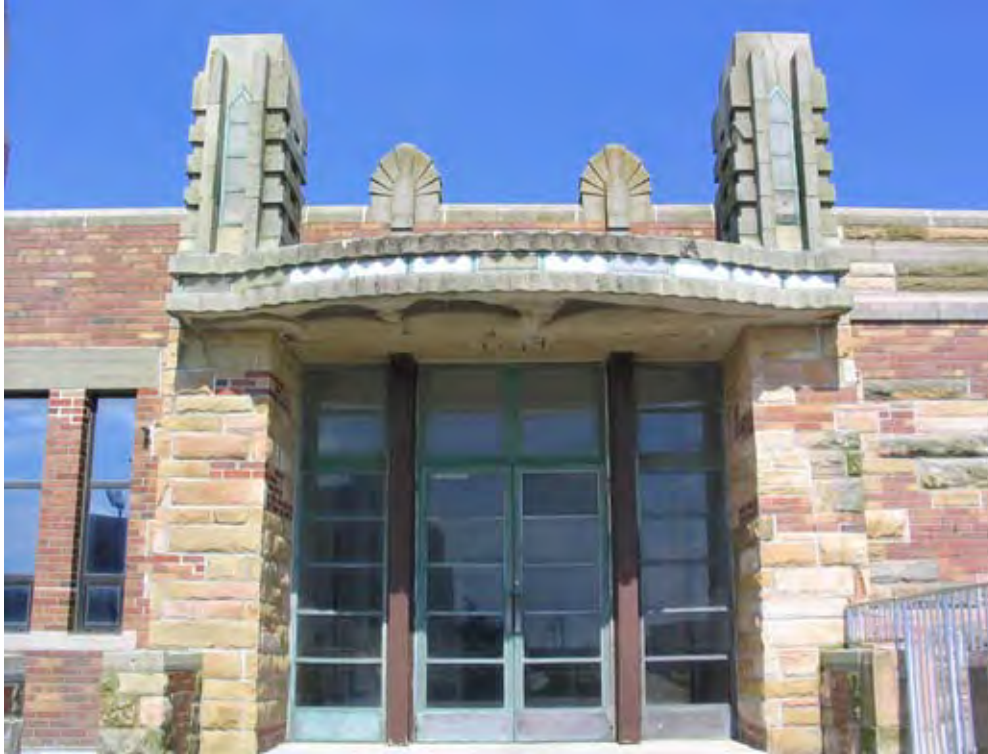
Figure 52: West Bathhouse west facade second floor showing original exterior metal doors, decorative glass, and cast-stone trim details at former Marine Dining Room entrance, 2004
