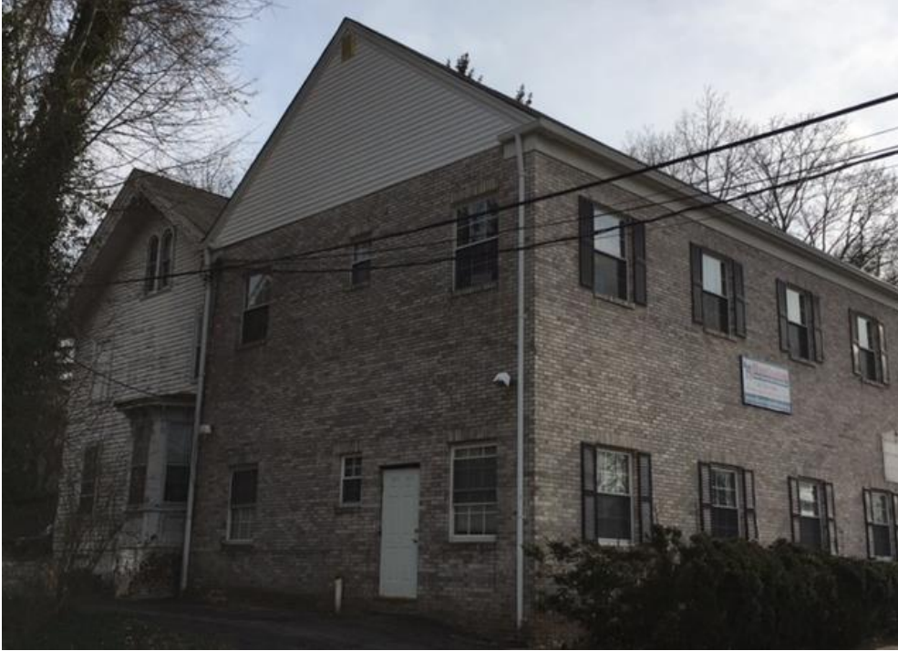
Addition in front of the historic house completely obliterates the historic house. Never a good approach.
