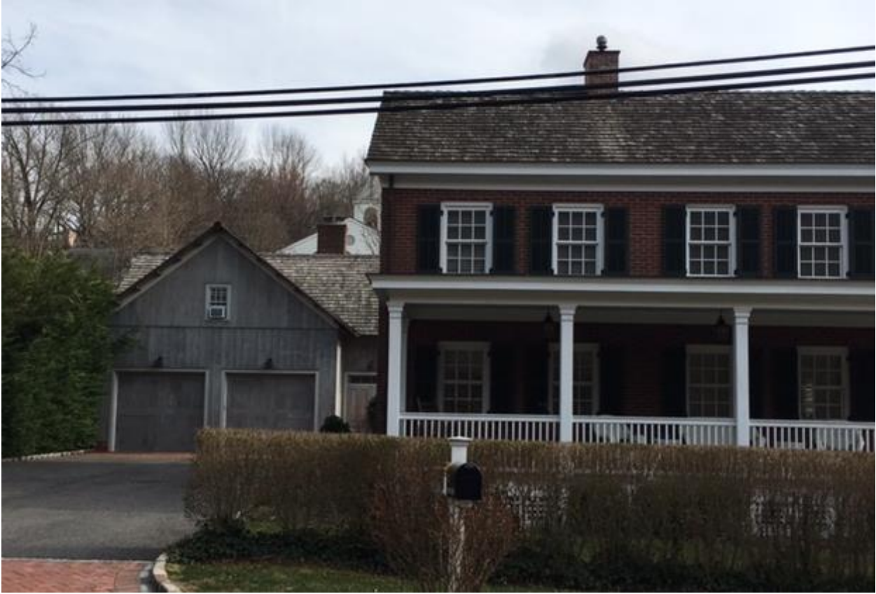
New garage is consistent in style and massing with what would have been built contemporaneously with the historic house.
