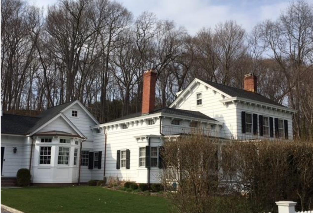
Addition to the side of the house is set back from the main block of the historic house.
