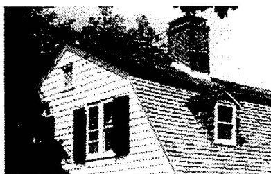
The gambrel roof is characteristic of Early English Style architecture.
