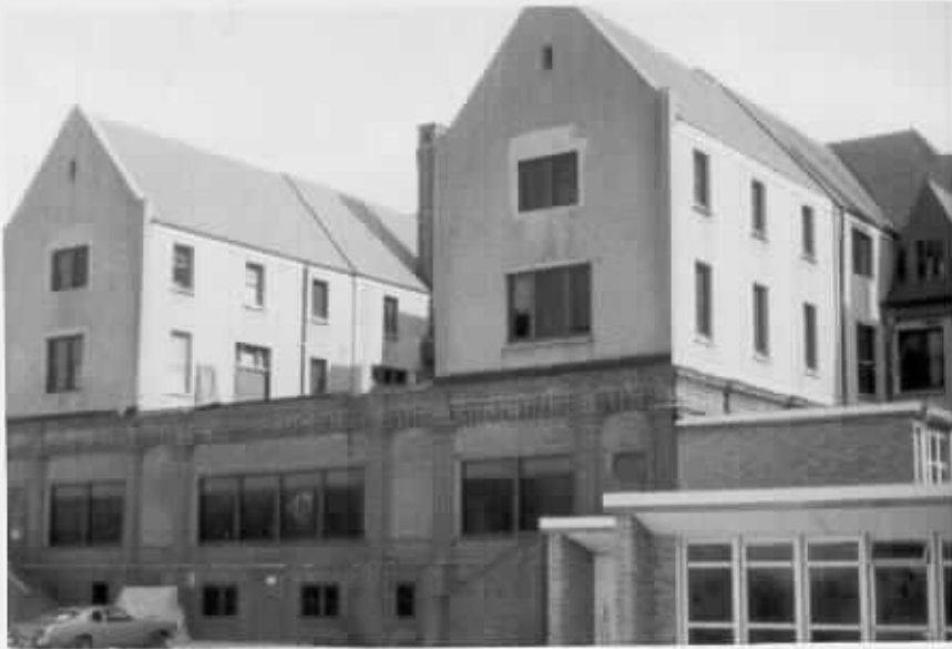
View of rear(north) showing additions
