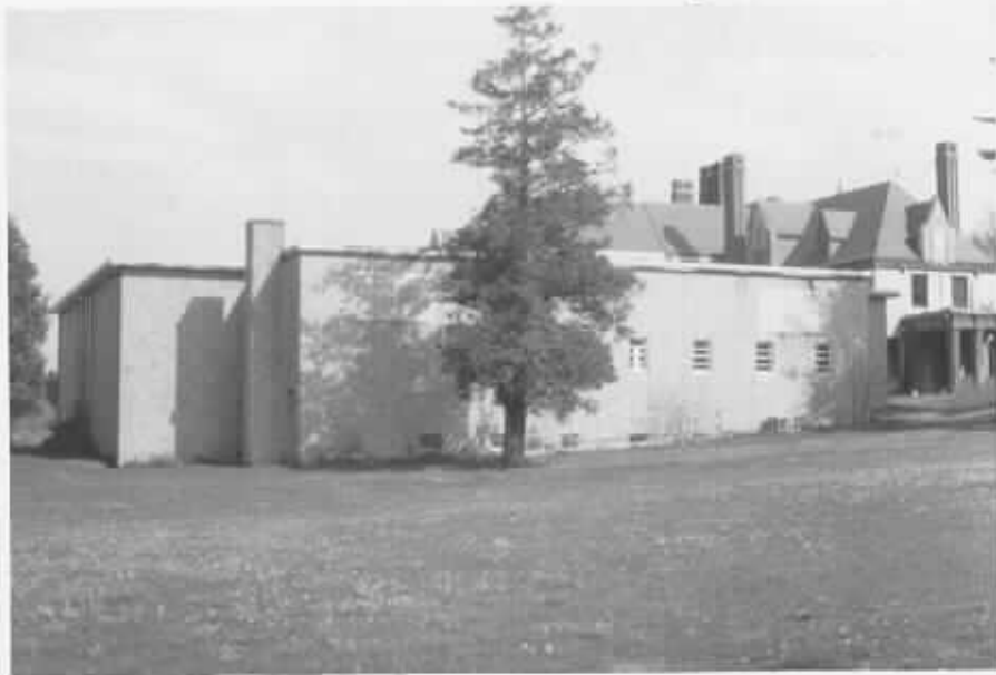
Addition at rear(north)
