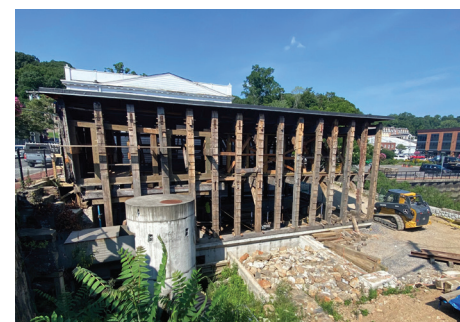
Roslyn Grist Mill lowered onto its new foundation. July 25, 2023.
