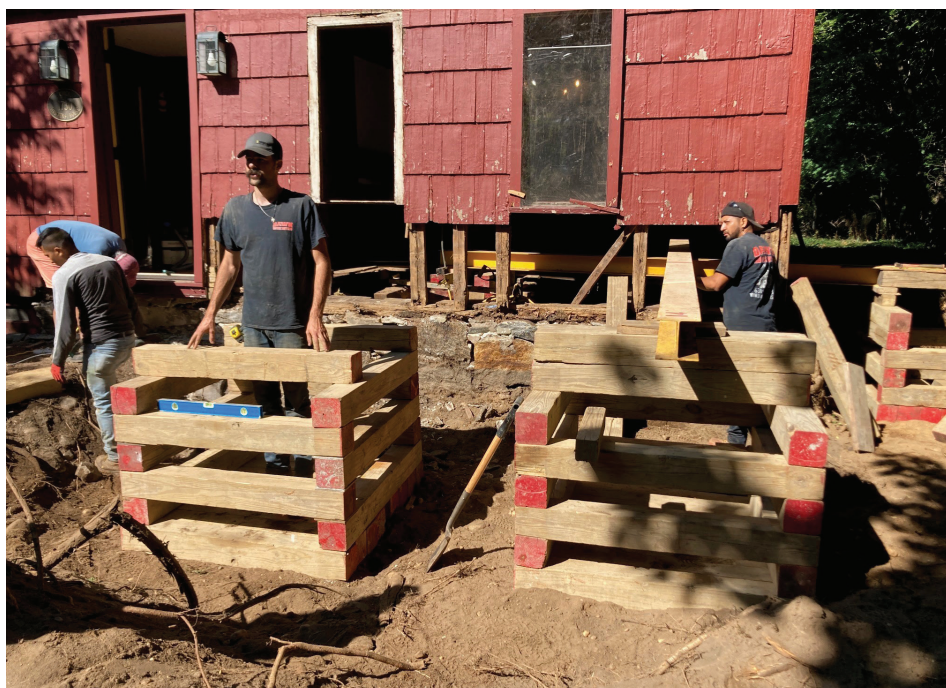
Workers laying a new foundation at the Hawkins-Elzon House. Courtesy Zach Studenroth.
